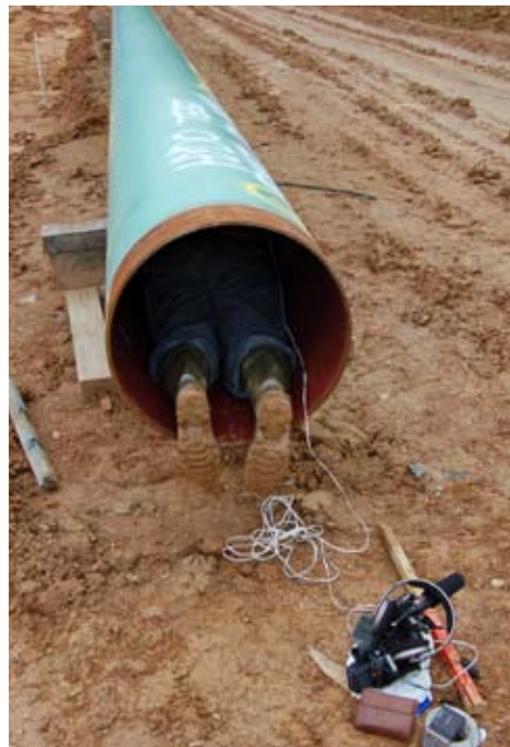
'Explaining Power to a Pipeline'
