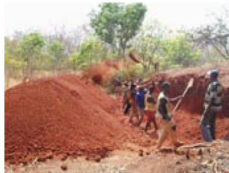
The project will rehabilitate 48 kilometres of road, enabling humanitarian aid to reach displaced populations in the Kabo region
