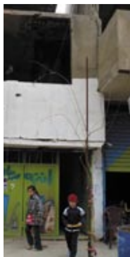
Salim's house after the first phase of repairs: 210 households have received the same kind of support so far in Nahr El Bared
